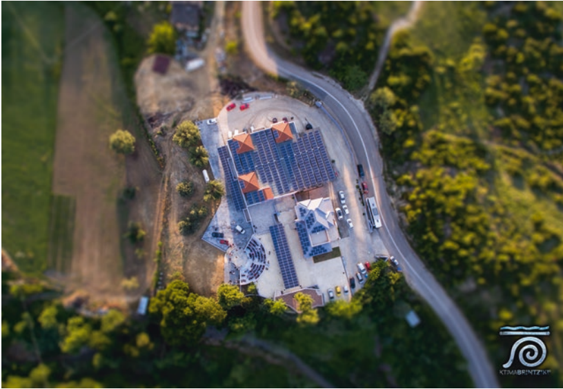
Fig. 17.4 Environment friendly: extensive use of photovoltaic panels and geothermy
